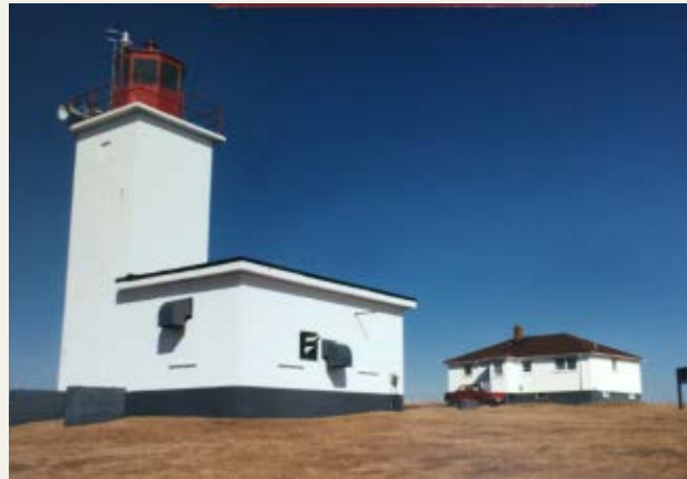
Replacement Lighthouse. Cap Sainte-Marie lighthouse and lightkeepers house. 1988. (Harold Robichaud)
